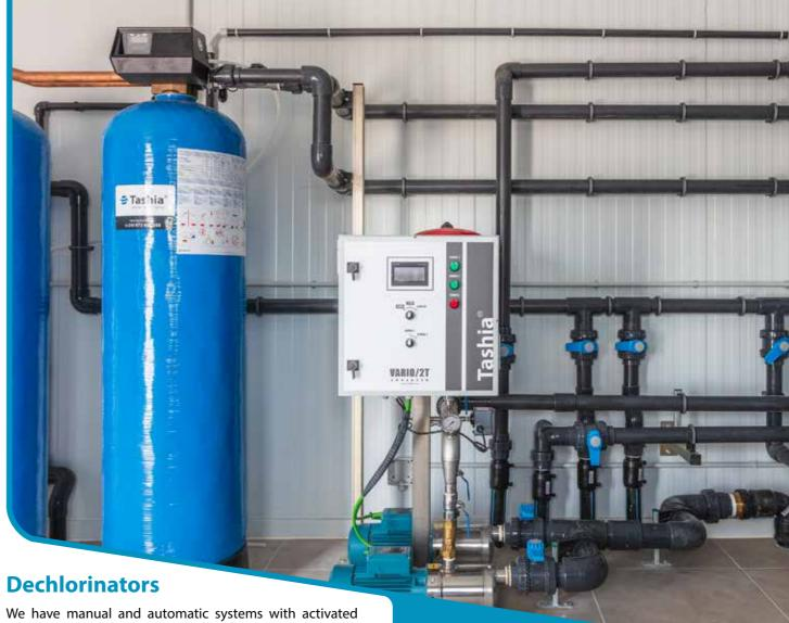
We have manual and automatic systems with activated carbon for the removal of free chlorine from water. It also has properties to remove organic pollutants, heavy metals, odors and tastes, etc.
